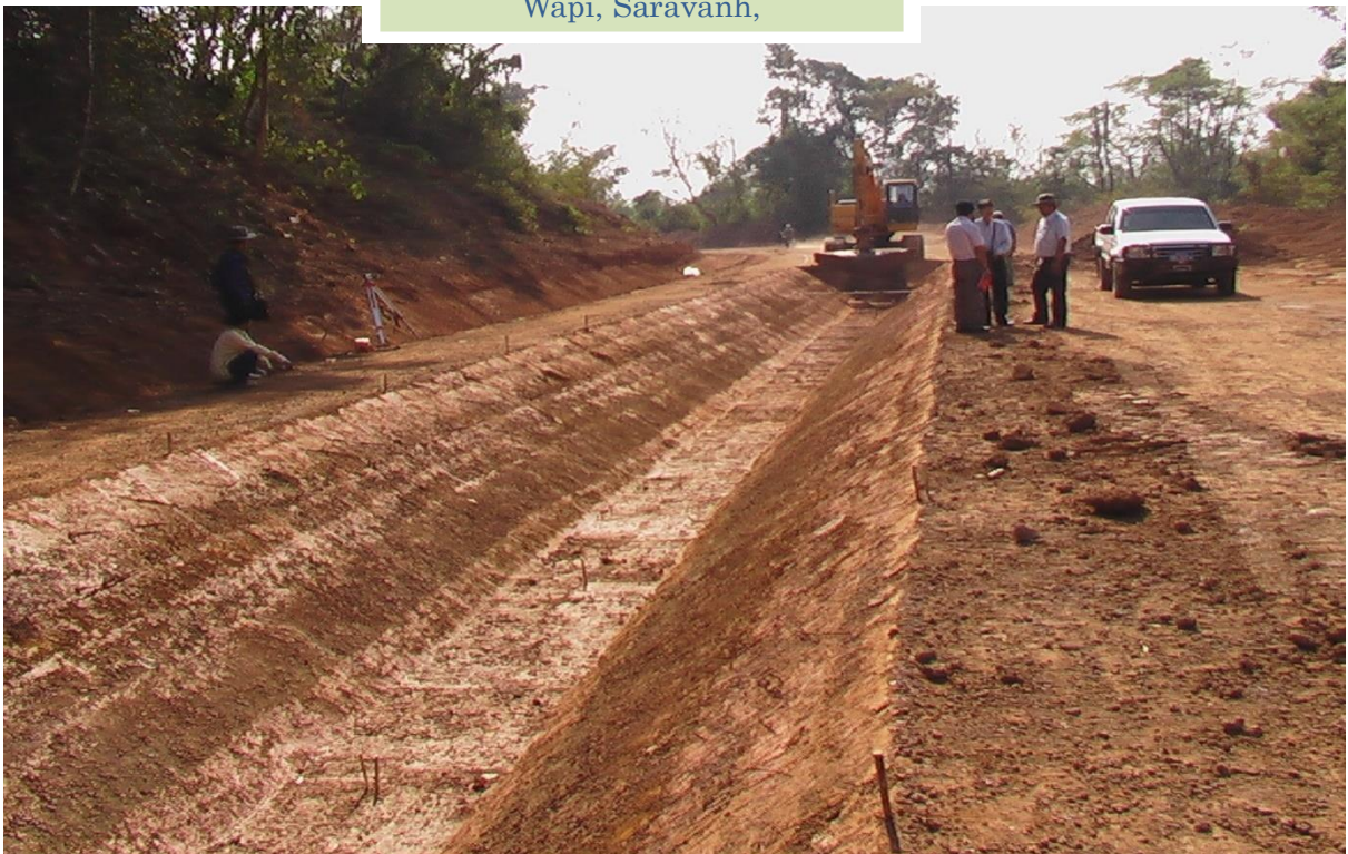
Irrigation construction supervision Wapi, Saravanh,
